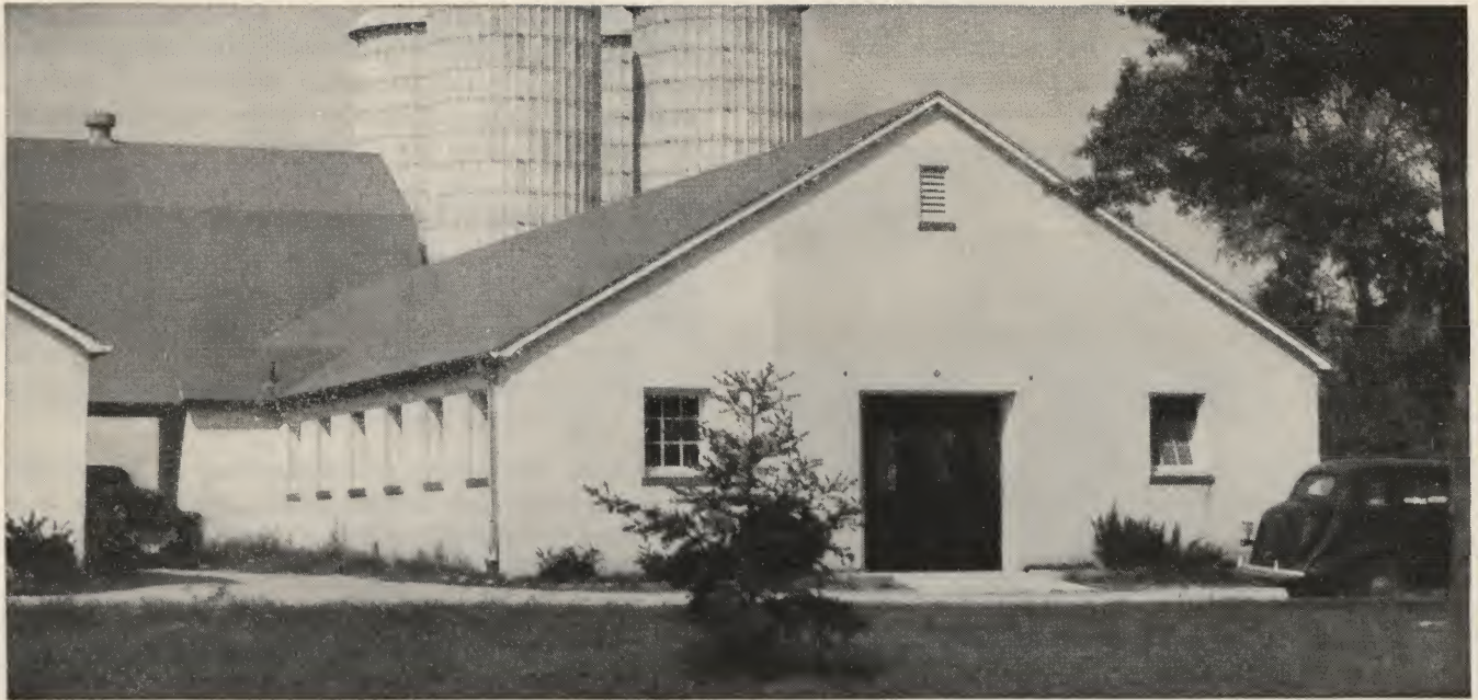
Attractive farm buildings of concrete block or concrete building tile are secured when a few simple rules of good concrete masonry construction are followed.
